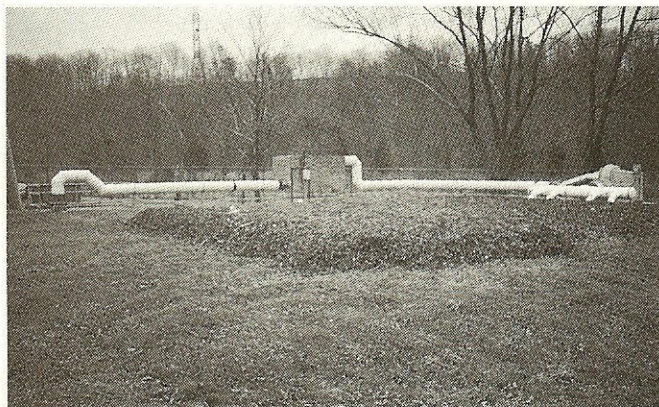
Compost biofilters remove a wide range of compounds at relatively high contamination rates.
