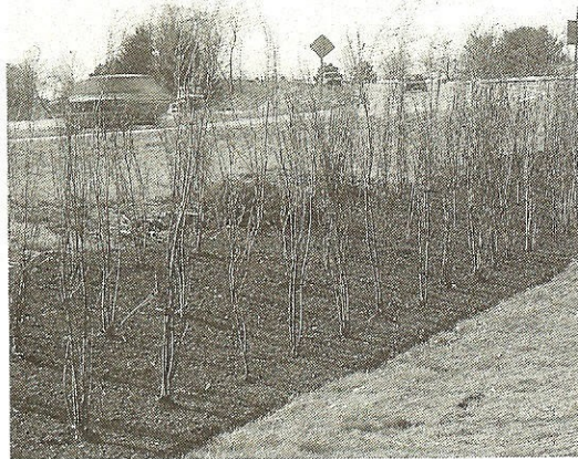
Compost berms at the base of slopes are very effective for erosion and sediment control.
