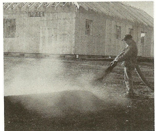
A pneumatic blower unit applies compost for establishment of a berm.
